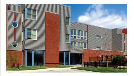
This project consisted of the construction of a new three story 17-unit apartment building, three new townhomes, and the renovation of nine apartments. The 17-unit apartment building was constructed to a LEED silver standard and entails a full vegetative roof systems, spray foam insulation, architectural metal siding, and brick veneer. Funded in part by the City of Philadelphia.
